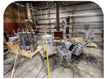
Figure 1. In the EPRI laboratory using reclosers provided by Avangrid, EPRI tested the ground reference of voltage sensors in steady state, during voltage steps and through temperature cycles to verify the measurement accuracy of magnitude and phase angle of the voltage readings.
