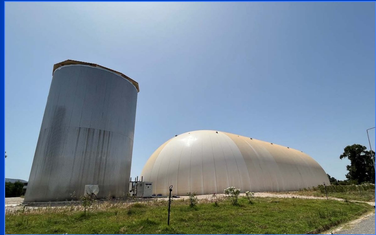
Figure 5. CO 2 Battery's Dome-Shaped Housing for the Inflatable Bladder Holding the CO 2 in Discharge Mode at Atmospheric Pressure (used with permission from Energy Dome)
