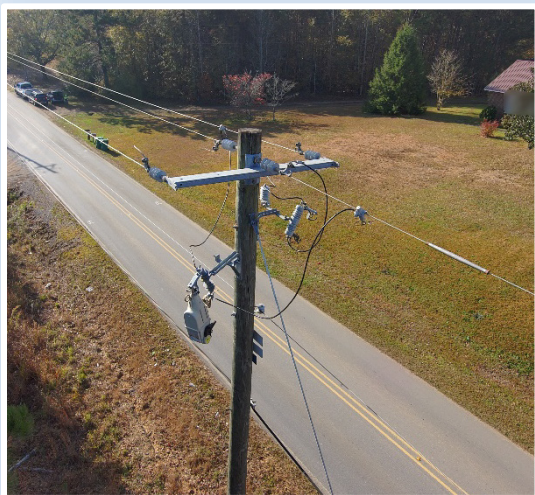
Example of a compact single phase recloser protecting a tap off the end of a three-phase line.
