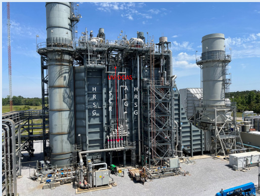
UV-DOAS NO x & NH 3 Measurements Between the Ammonia Injection Grid (AIG) and SCR Catalyst
