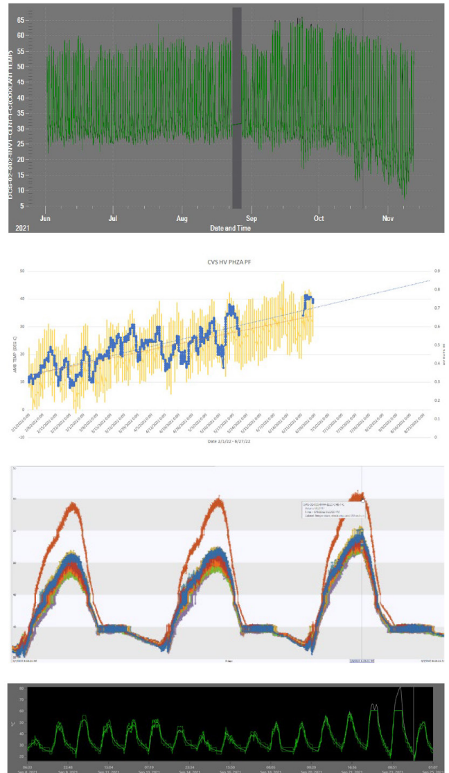
Figure 4. Tracking temperatures of different components of the central inverter of a utility-scale PV plant through SCADA
