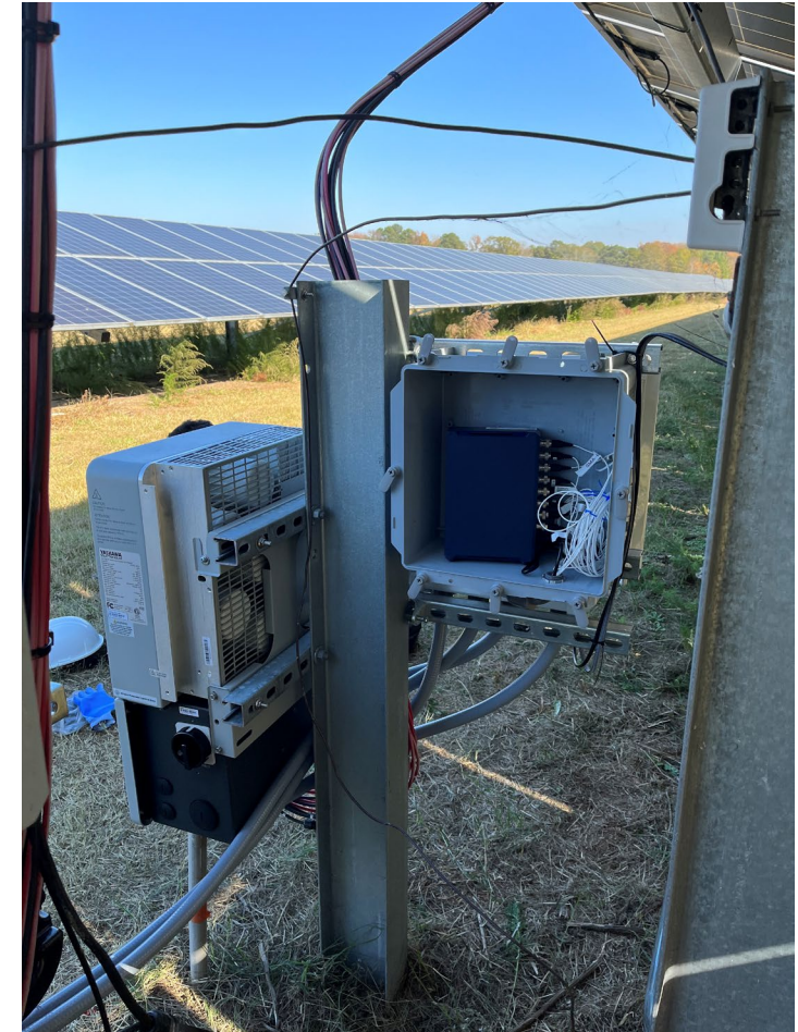
Box with amplifier can amplify the signal from the installed high frequency microphones before sending it to data box
