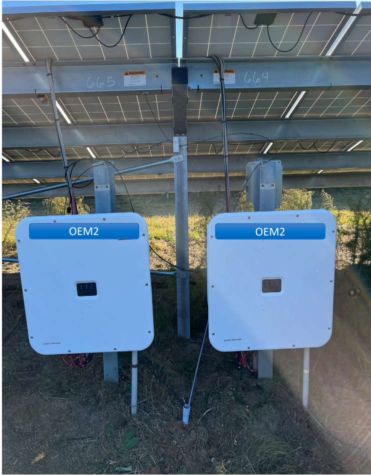
Repowering with OEM2 inverter
