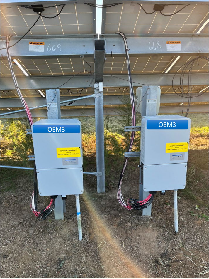
Repowering with OEM3 Inverter
