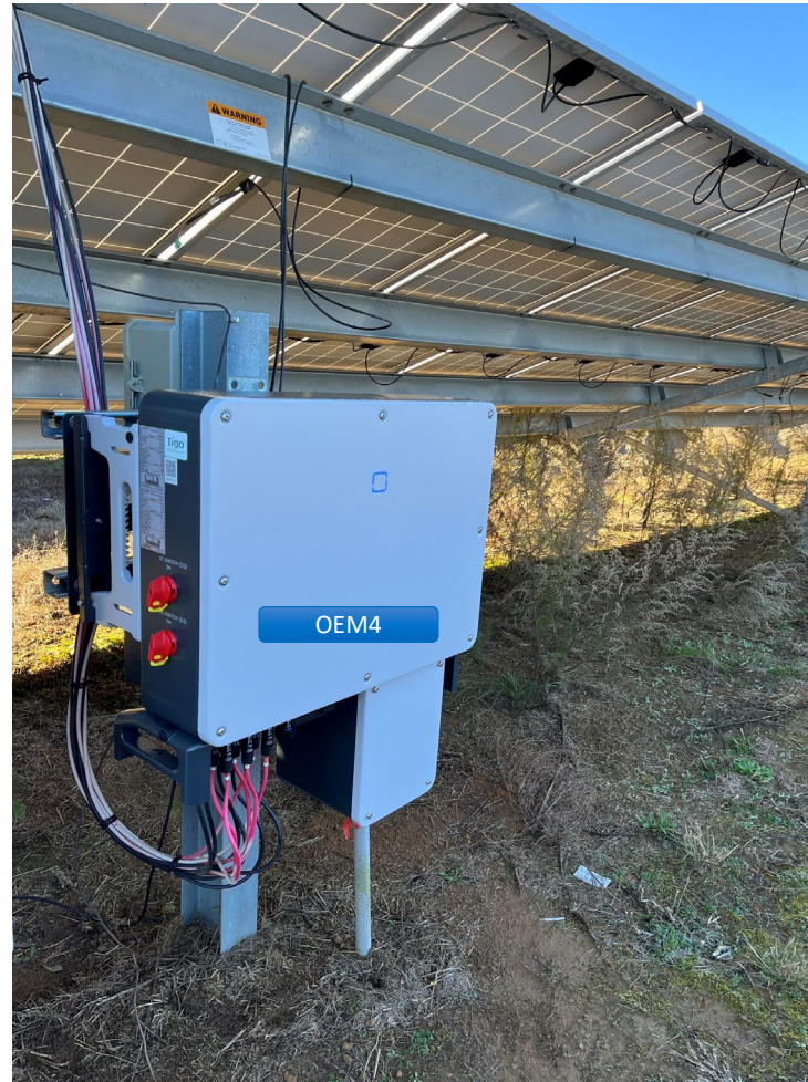
Repowering of OEM3 and OEM4 inverters pair
