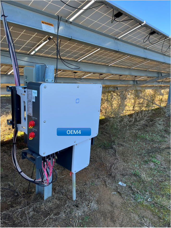
Repowering with OEM4 inverter
