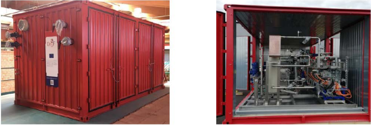
Figure 3. Exterior and Interior Views of Heat Pump used at Wienerberger Uttendorf (Schneeberger et. al)
