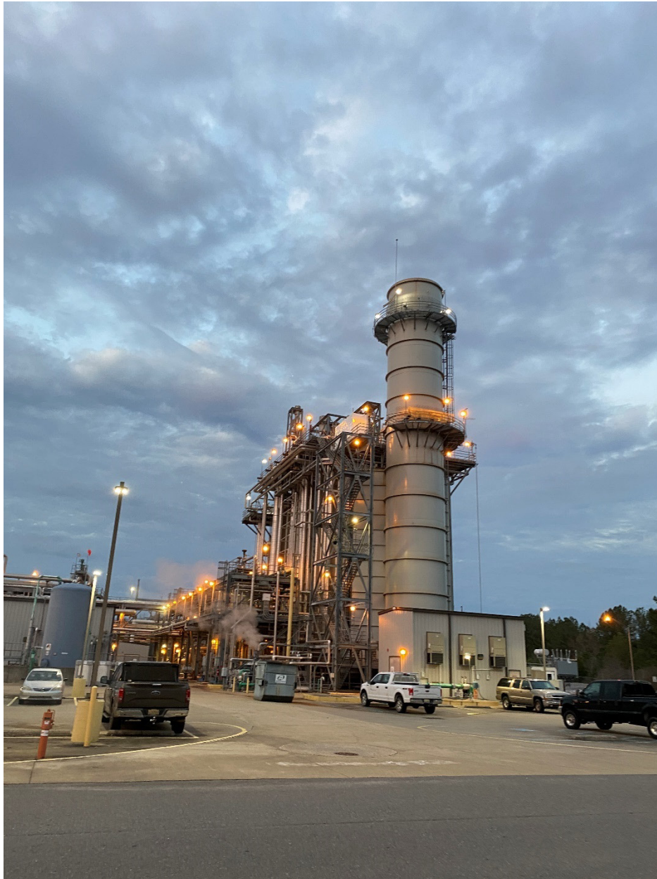
Figure 3 Hillabee Generating Station
