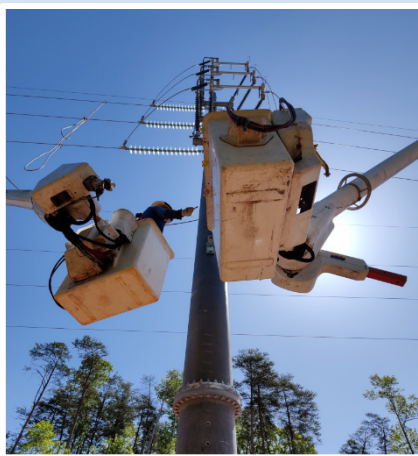
Line switch inspection
