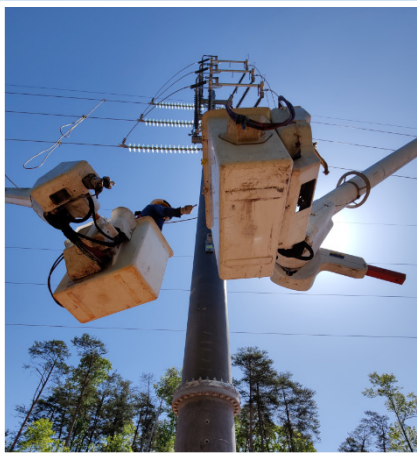
Line switch inspection
