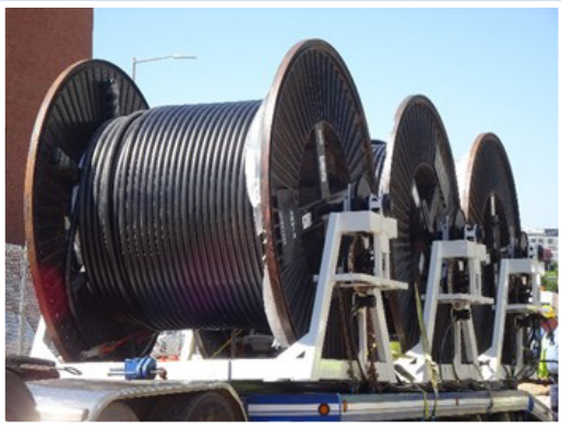
Extruded pipe-type cables
