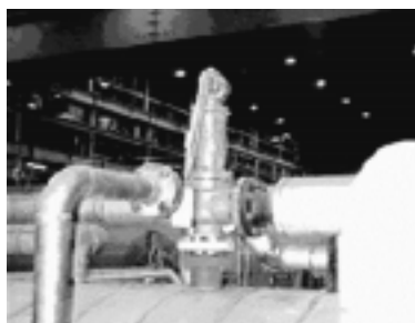
Figure 41: Visual Feedwater Heater Relief Valve
