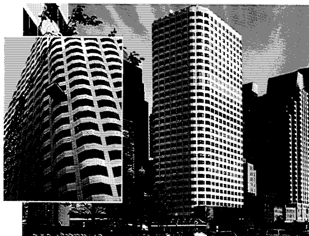
Figure 1. Chiller installation at 99 High Street.
