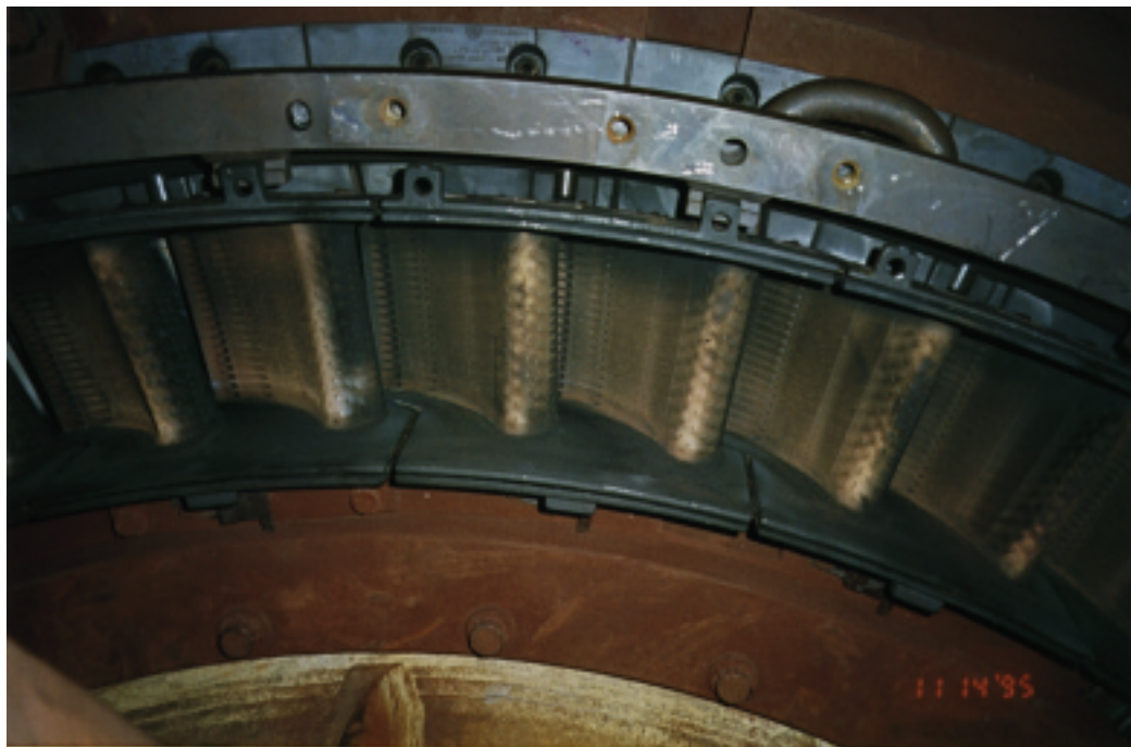
Figure 8.17 Unit 4B 11/95, 14,264 hrs. 3rd Stage Buckets.
