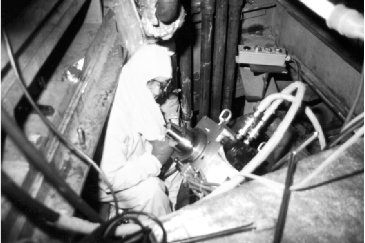
Figure 6-8 Valve Body Machining
