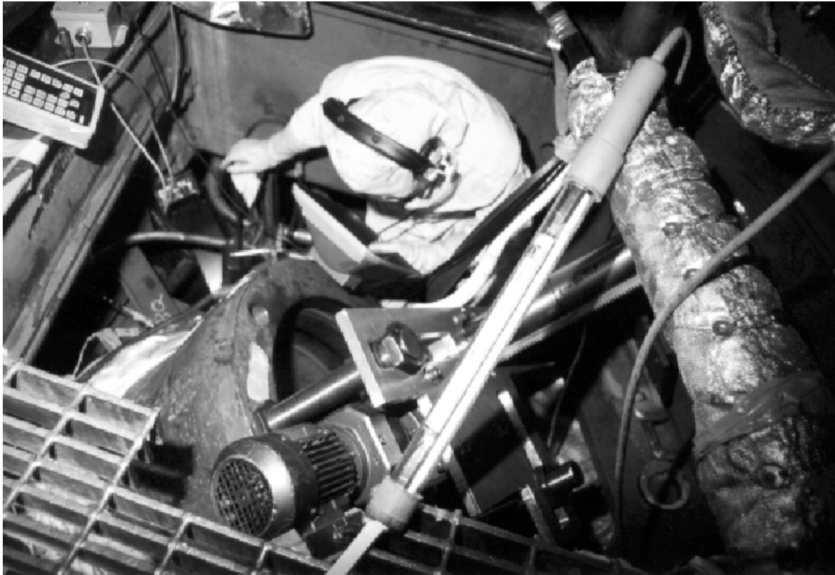
Figure 6-6 Welding At Valve
