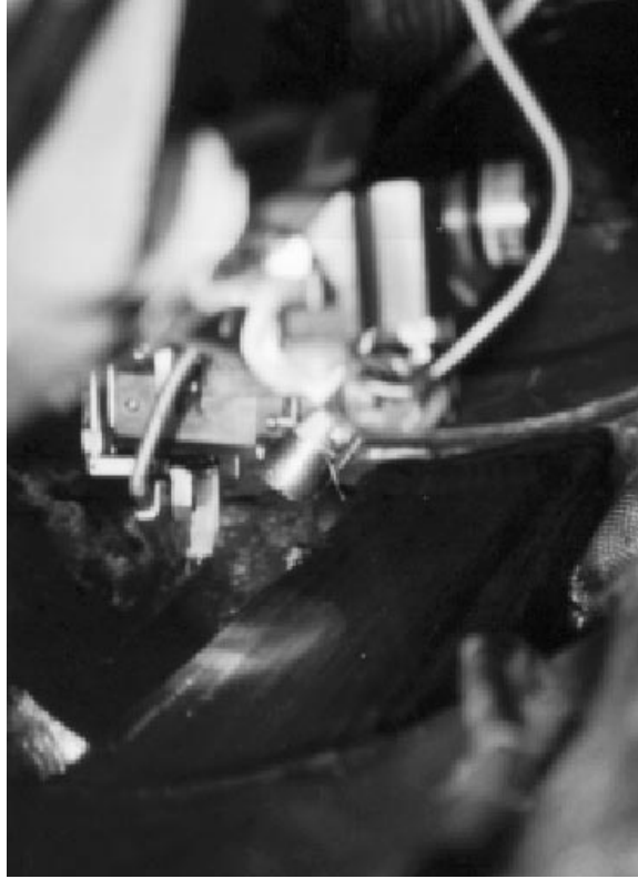
Figure 6-7 Welding Inside Valve
