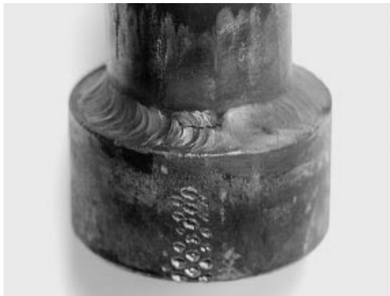
Figure 3-4 Fatigue-Induced Crack in Socket Weld
