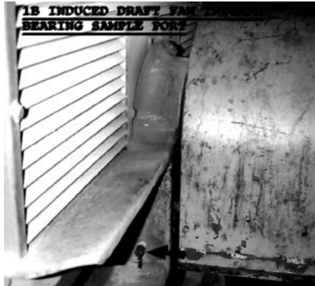
Figure 3-13 Sampling from Sample Fitting - Journal Bearing
