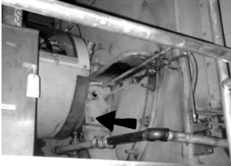
Figure 3-10 Sampling from Oil Sample Fitting
