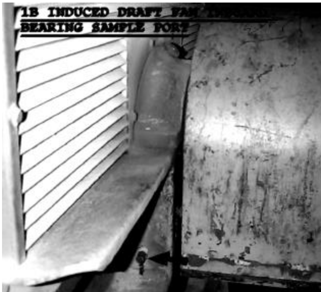
Figure 3-13 Sampling from Sample Fitting - Journal Bearing
