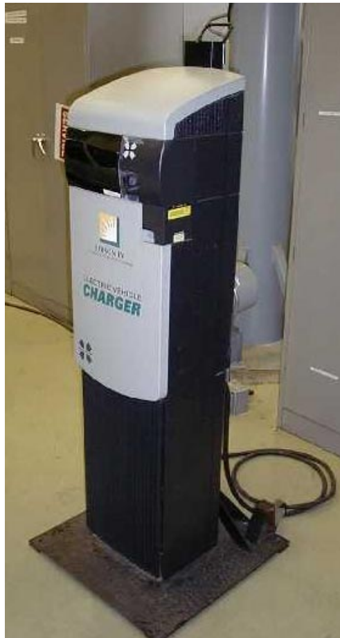
Figure 3-1 Hughes 6.6 kW Gen I Inductive Charger
