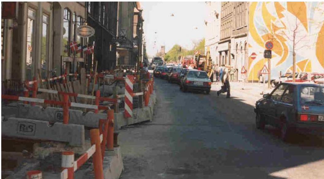
Figure 7-1 Typical Open Trench Barriers in Copenhagen
