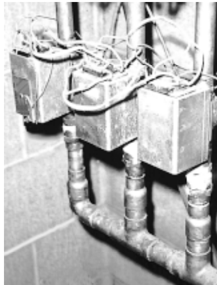
Zone valves, powered by a 24-volt control circuit, provide on-off flow control using a single circulator.
